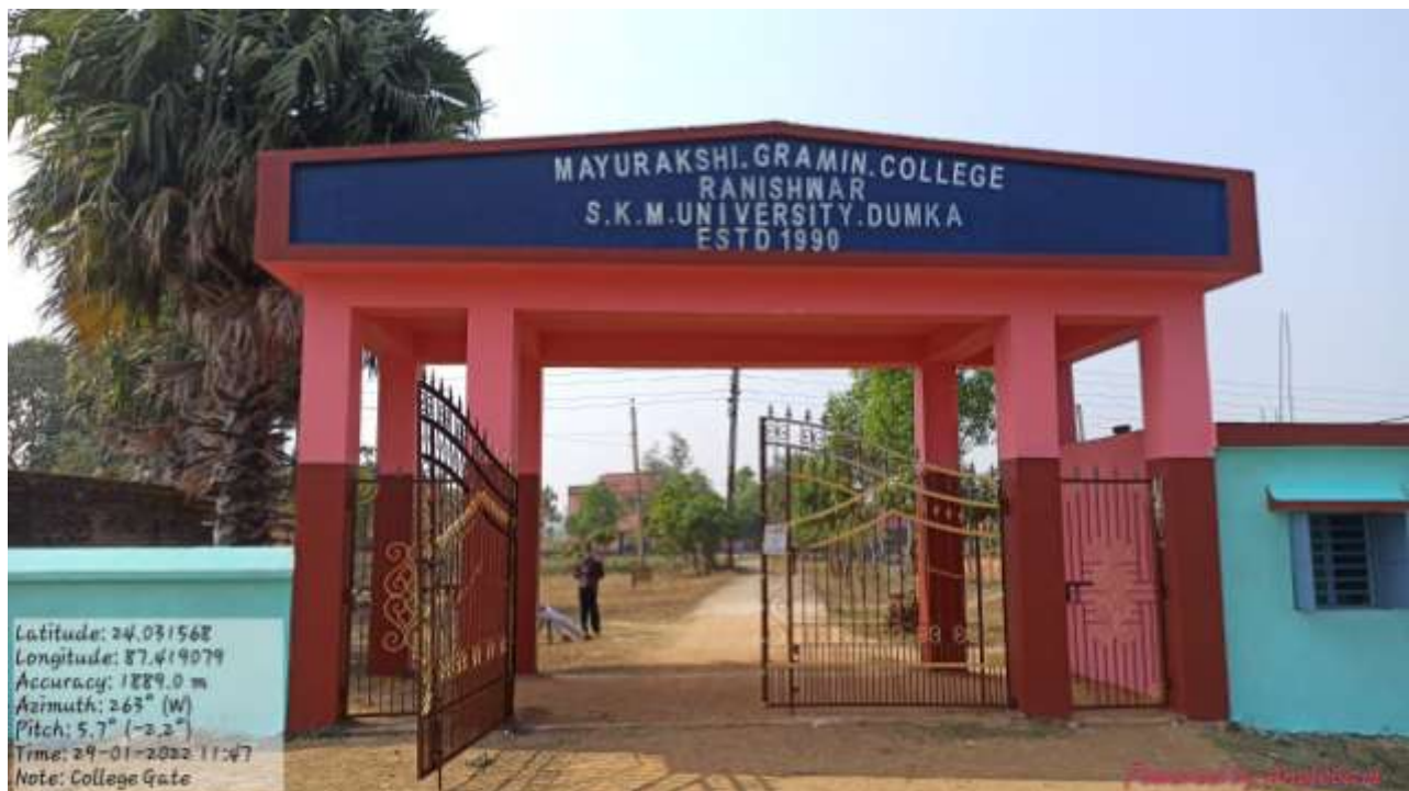
Figure 4: Restricted entry and secure campus.
